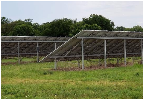
Example of a Solar Conversion System, Ground-mounted
